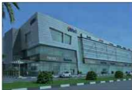
Eiffel Buildings Dubai - U.A.E.
