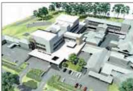
Kempsey District Hospital Kempsey - Australia
